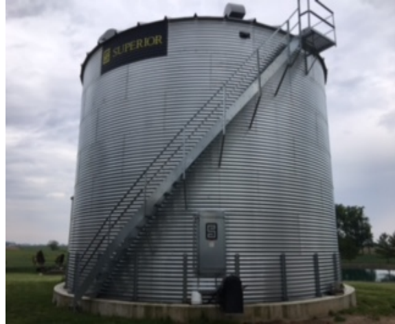
Grain bin with steps and guardrails
